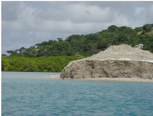
Figures 7 and 8: Placement of fill without appropriate mitigation to prevent runoff (left), soil slumping and siltation has resulted in severe increases in turbidity to the near coastal waters (right).
